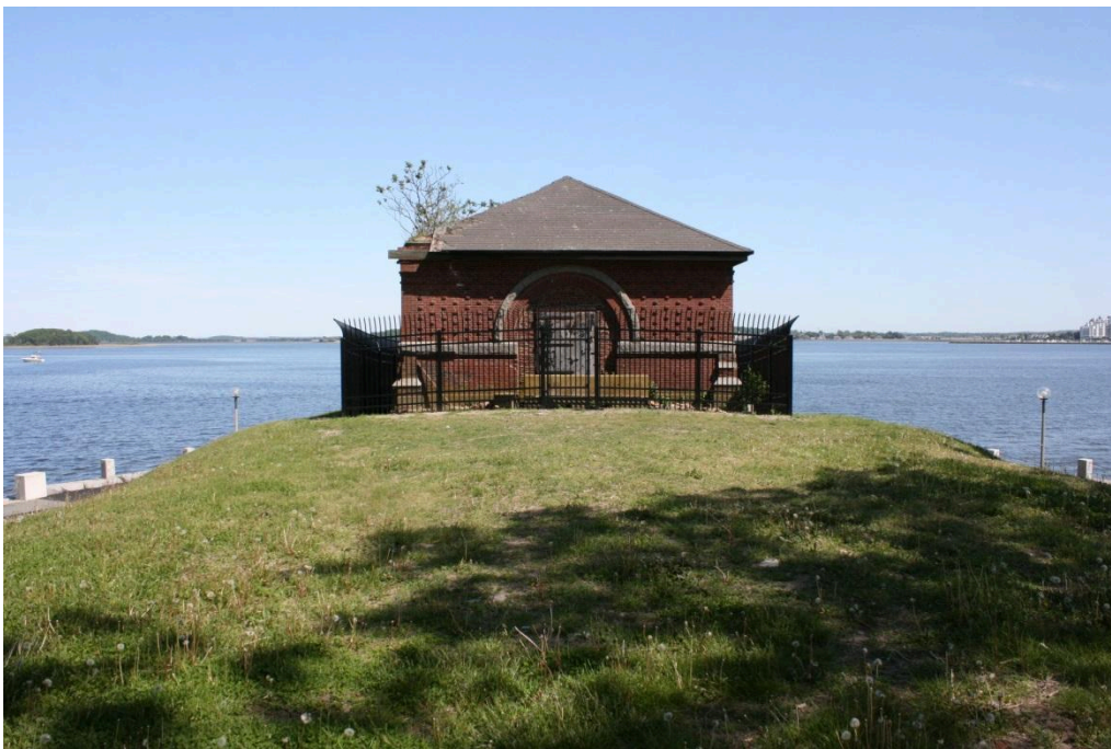
Figure 12. West Shaft Entrance.
