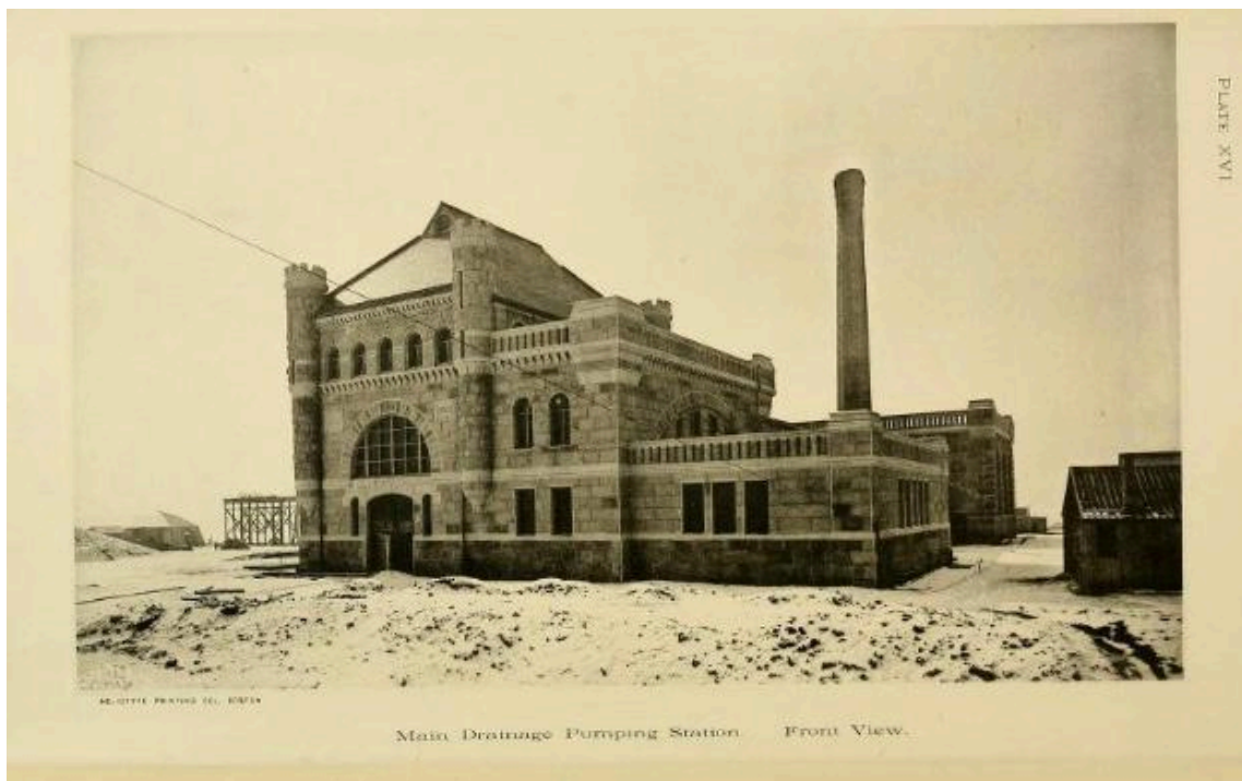
Figure 17. View of the front of the Pumping Station Source: Clarke, Eliot C. Main Drainage Works of the City of Boston. Boston: Rockwell & Churchill, 1888.
