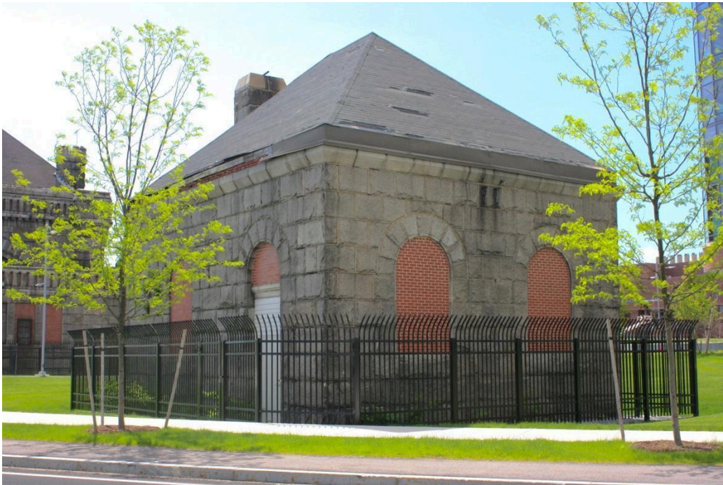
Figure 10. Gate House/Filth Hoist.
