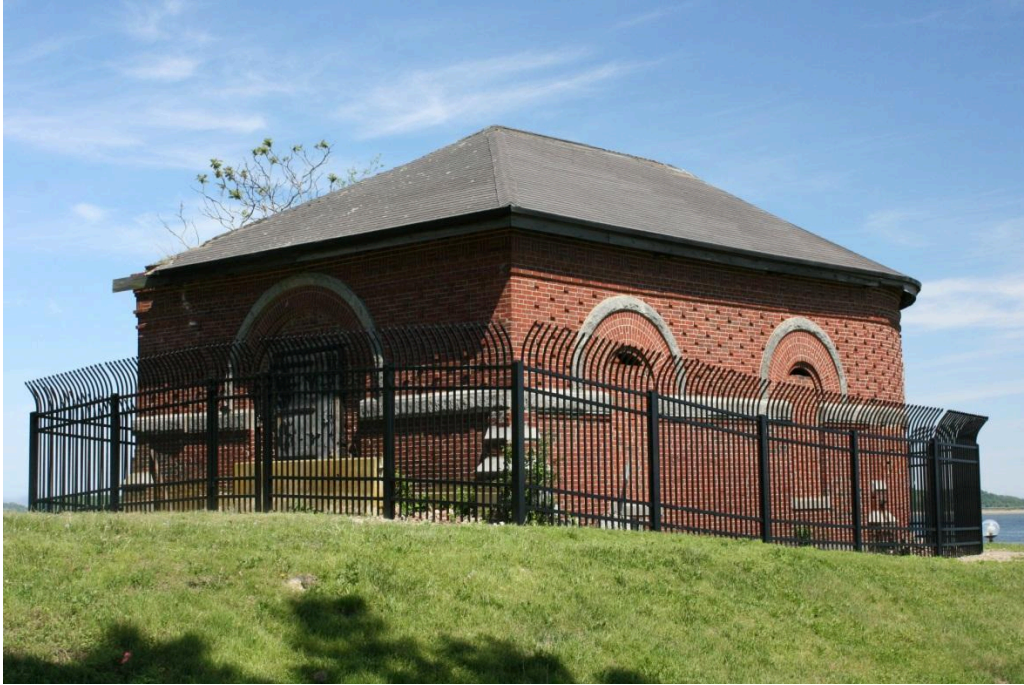
Figure 13. West Shaft Entrance.
