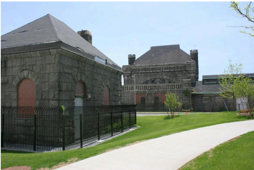
Figure 8. Gate House/Filth Hoist and Pumping Station.
