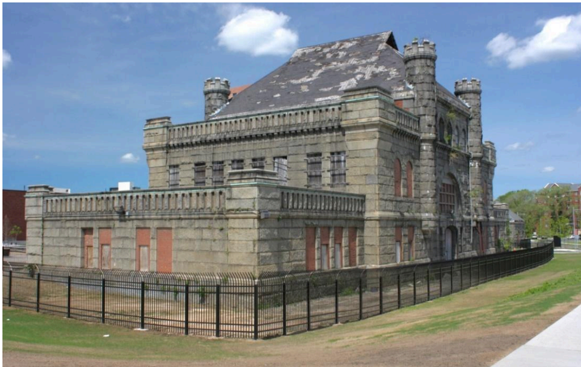
Figure 2. Pumping Station: Engine House.
