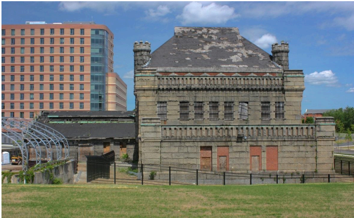
Figure 6. Pumping Station: Boiler House and Engine House.
