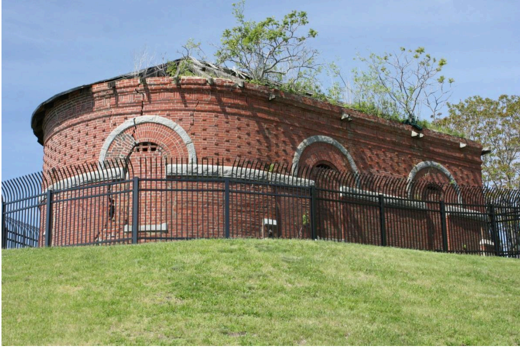
Figure 15. West Shaft Entrance.
