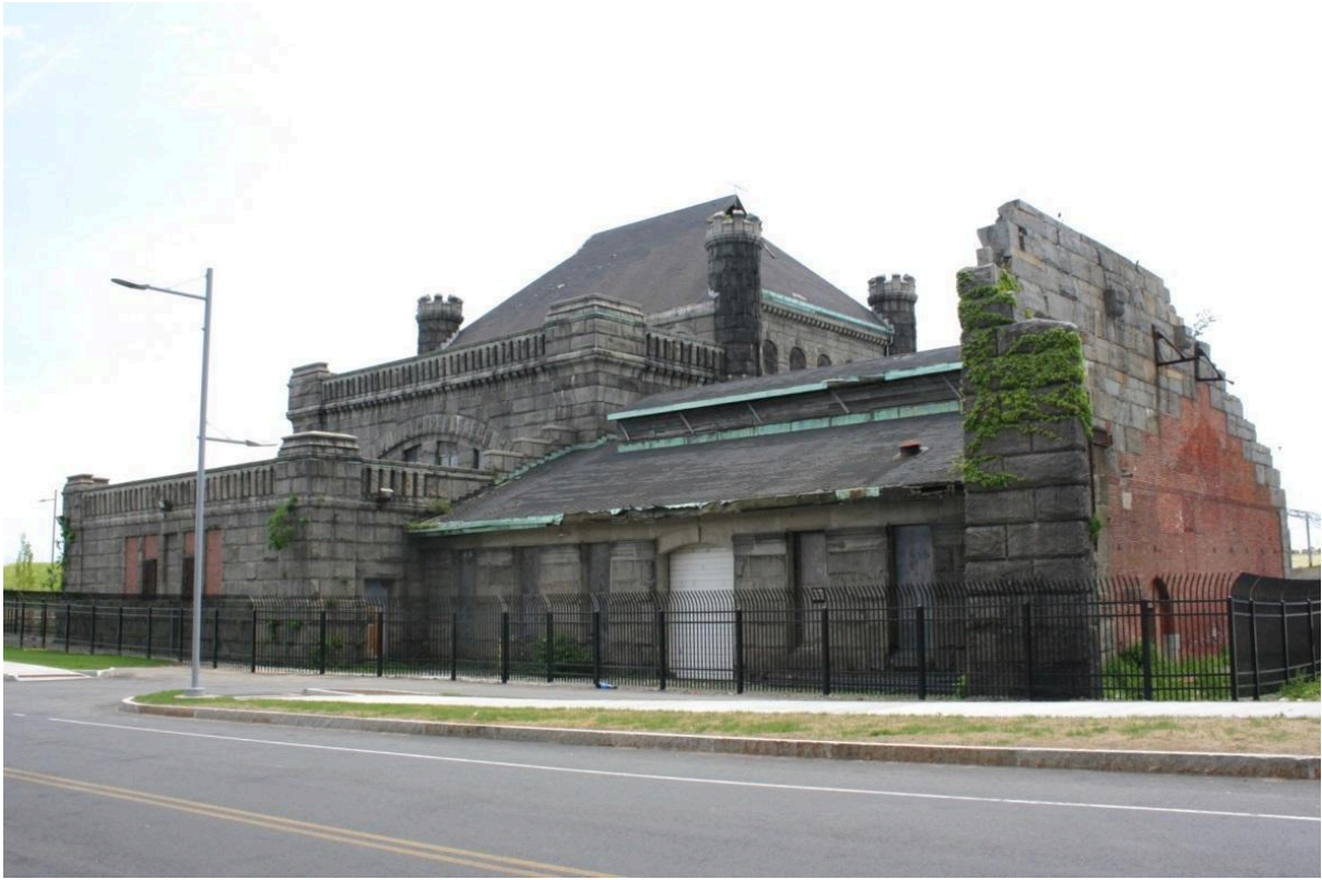
Figure 4. Pumping Station: Engine House and Boiler House.
