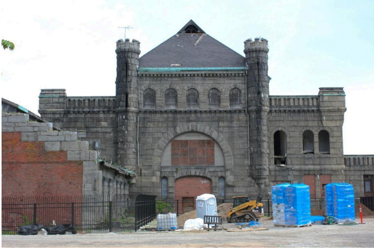
Figure 5. Pumping Station: Boiler House and Engine Room, rear elevation.
