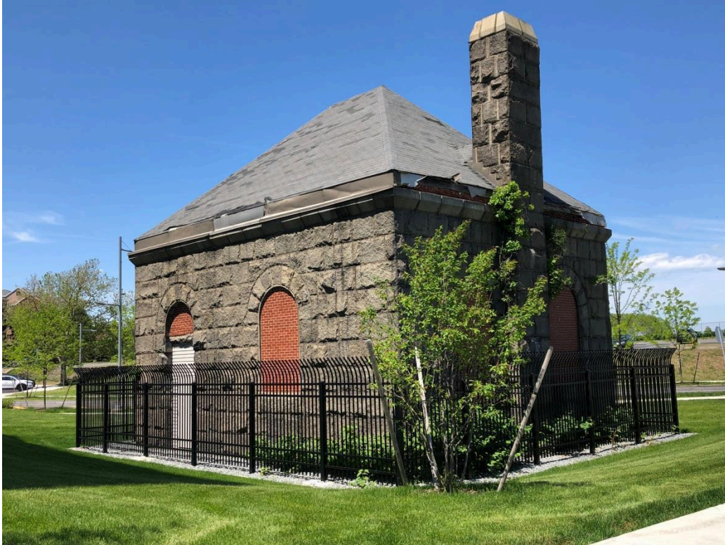
Figure 9. Gate House/Filth Hoist.
