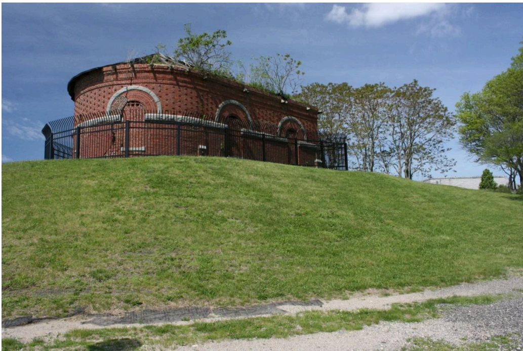
Figure 14. West Shaft Entrance.
